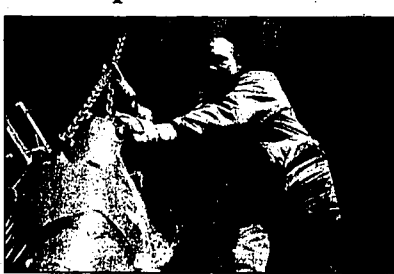
Burley city worker Eliseo Haro guides a pump through the roof of the sewer pumping station at Fifth Street and Hilland Avenue. Two pumps were replaced because replacement parts were becoming hard to find. Some parts were broken when sheets and uniforms flushed down toilets clogged the pumps.
