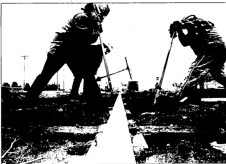
Doug Keiley, left, and Ron Setser, right, hold a rail and railroad tie in place while Daniel Beltran pounds a spike in place on a rail siding in Kimberly. The rails were warped in the intense heat of a warehouse fire on October of 2001. Several sections of charred ties have to be replaced, as well as the rails, before the track can support heavy rail cars again.
