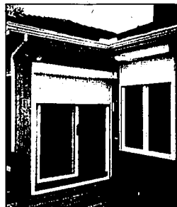
Rolling shutters can be installed over windows or sliding glass doors.
