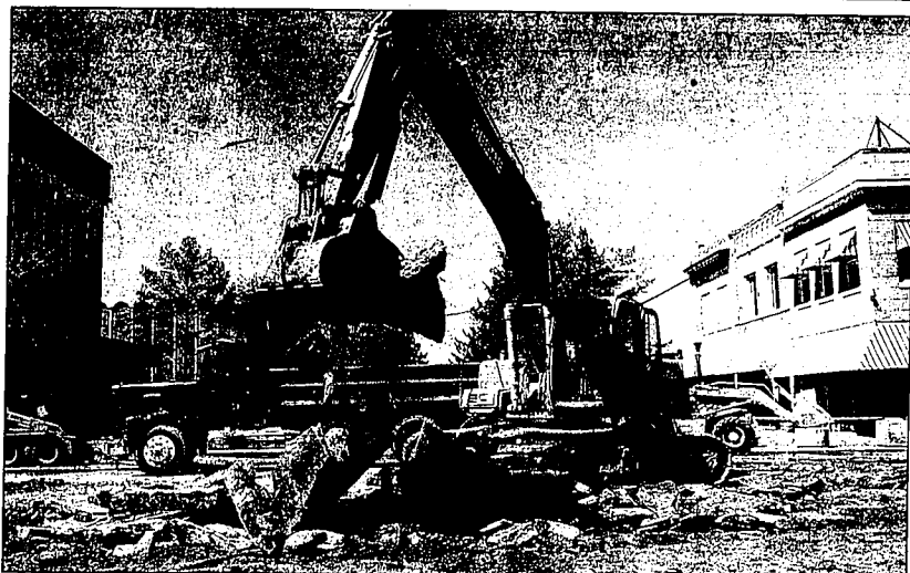
A trackhoe loads broken pavement onto a dump truck at the intersection of Shoshone Street and Main Avenue in Twin Falls Tuesday. Crews will be working to install new pavement for about a month.
