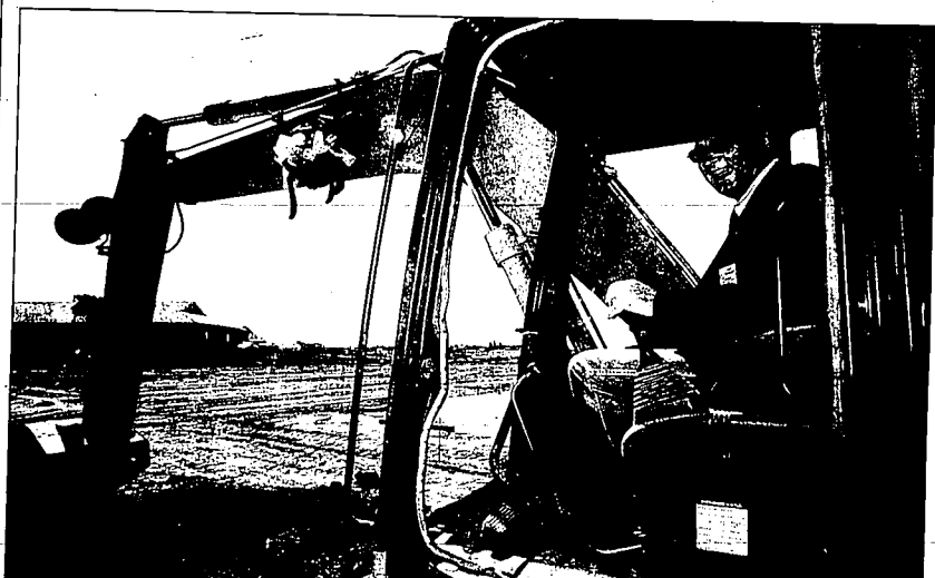
Twin Falls County Commissioner Gary Grindstaff uses a track hoe to officially break ground on a new building for the South Central Community Action Agency in Twin Falls on Friday.
