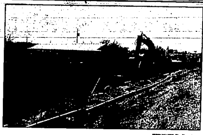
Work on a new sewer system for the city of Paul began the first of the month. The initial work is occurring near the railroad tracks and the elementary school.
