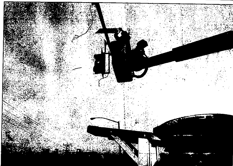
George Dalns lifts a 'Left Turn Only' sign off a traffic light at the intersection of Blue Lakes Boulevard and Pler Avenue in Twin Falls. The Idaho Transportation Department replaced the old style lights with 'permissive' left turn indicators. The new lights will allow motorists to turn left when the light is green for through traffic after they have yielded.
