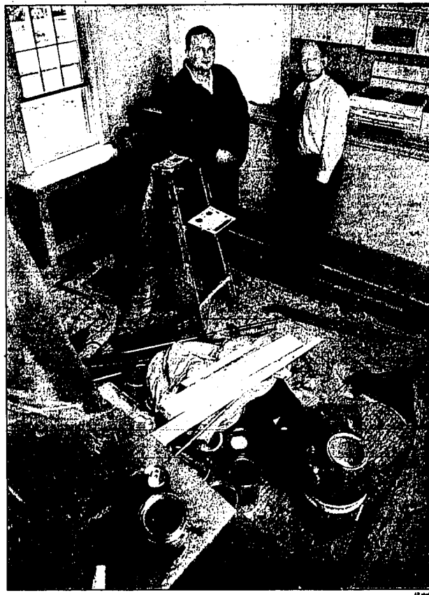
Homeowner Kenneth Chamlin, right, stands in his Ocean Township, N.J., home with his contractor, Keith Kinsey, while Kinsey's employee, Scott Charlier, does electrical work Tuesday.
