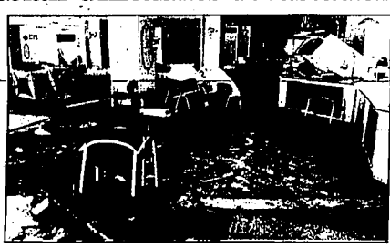
The damaged beachfront restaurant of the Sonesta Beach Resort is pictured Saturday in Southampton, the day after Hurricane Fabian hit Bermuda.
