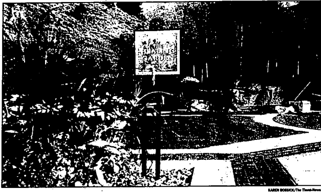
A worker applies the finishing touches to the new Healing Garden at St. Luke's Wood River Medical Center. A special presentation involving labyrinths and featuring a moment of reflection for the events of 9-11 will be held on Thursday.
