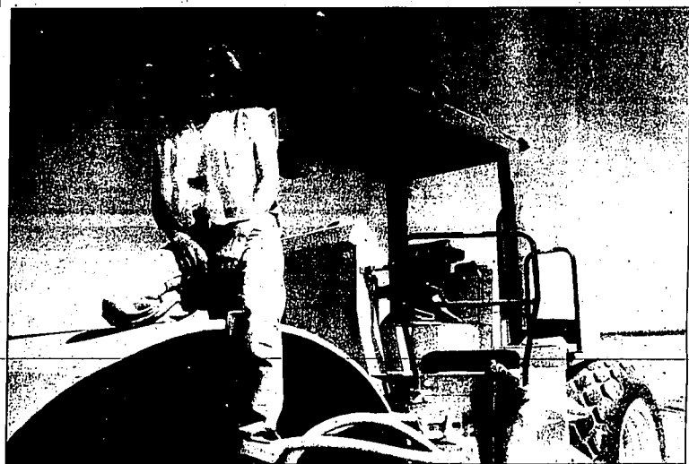
Janan Edwards, of Blackfoot, sits atop a steel-wheeled roller Wednesday in Glens Ferry. After completing a five-week course in Pocatello, Edwards began working on the King Hill freeway project in July and has been operating the machine there ever since.
