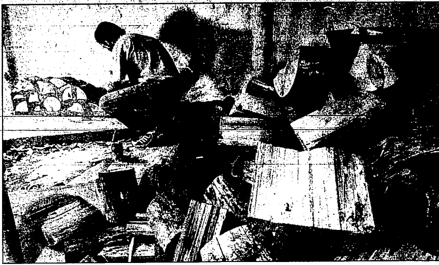
Alan Stankevitz uses short cedar and red pine logs to construct an interior wall in the cordwood house he is building in La Crescent, Minn. He has spent five years building the house by himself out of cordwood, a material most often used for firewood.
