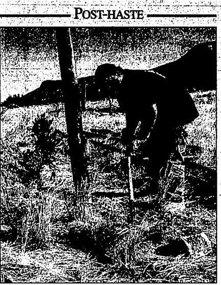
Albion resident Gary Clark installs posts for a fence he's building around his family property on Idaho Highway 77 in Connor Creek.
