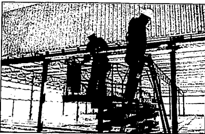
Workers from Mountain States Steel Erectors of Bigham City, Utah, prepare to install girders that will support the storefront frame of the new M.H. King's store being constructed at U.S. Highway 30 at the east end of Buhl.
