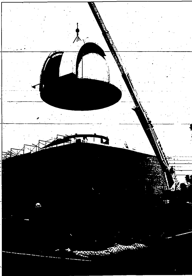
Workers hang on to several guy lines while the new observatory dome is lifted atop the roof of the Herrett Center for Arts and Science Saturday. The dome will house a custom-designed, research-grade telescope that will be fully hand-capped accessible. Once it is completed, the telescope will be open to the public as well as research.
