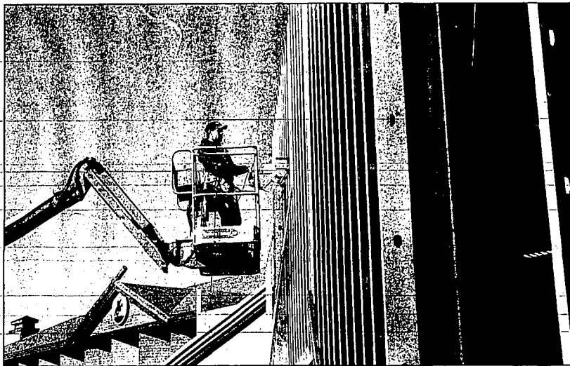
Larry Karvoski of Drywall Specialties out of Spokane, Wash., works on the expansion of The Coeur d'Alene Casino in Worley on Nov. 13. At a remote crossroads east of Spokane, the Coeur d'Alene Indians have taken control of their economic destiny. The tribe's decade-old casino is thriving. With a new 18-hole golf course, and an expanded hotel and casino under construction, the complex near the intersection of U.S. 95 and Idaho Highway 58 is closer to becoming the destination resort the tribe envisions.
