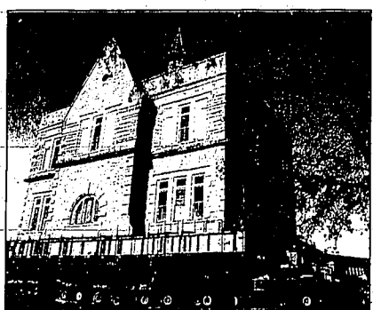
Crews from Lindsay Moving of Seattle move the Oneida Stake Academy in Preston, Wednesday. A group of volunteers dedicated to restoring the Latter-day Saints Academy raised more than $4 million to help move the building from a high school campus to a local park, three blocks away.
