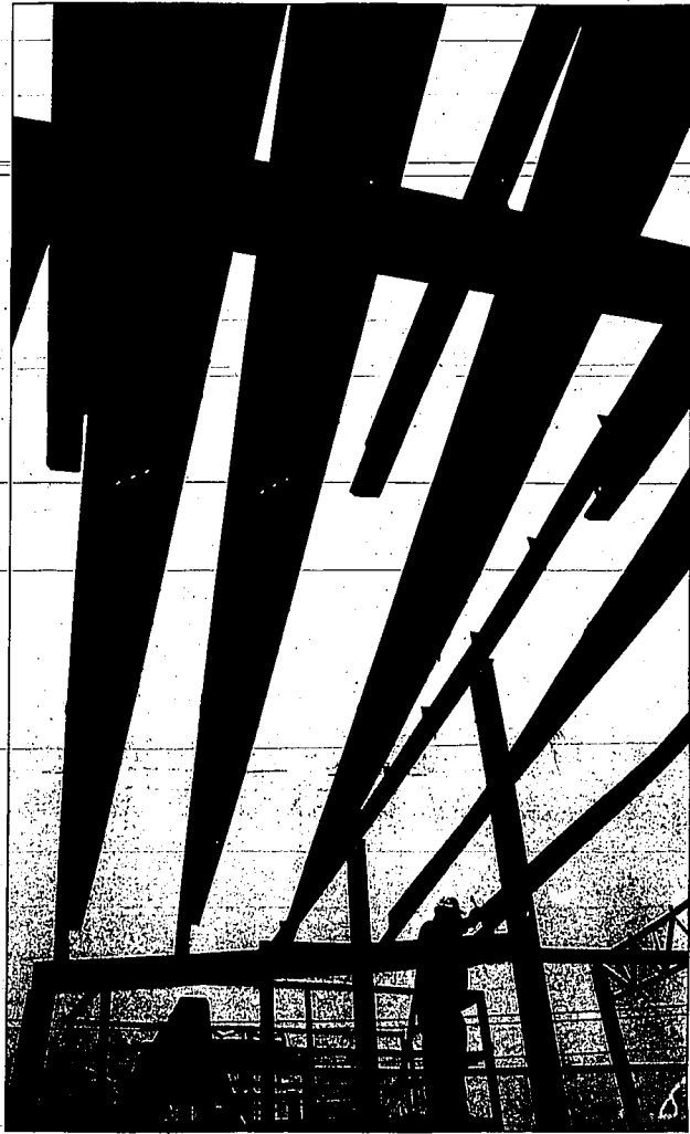
Jose Meraz tightens bolts on steel beams on a new industrial spec warehouse and office in the Intermodal area southeast of Twin Falls.
