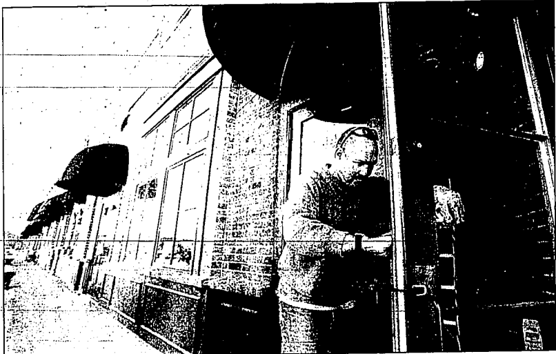
Ketchum carpenter Hank Balmer attaches door hardware at one of the new shops at the Bullion Square shopping center. He has worked on the Hailey mall project since May.
