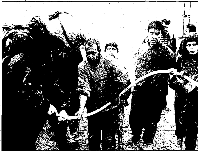
A U.S. soldier helps Iraqis install running water in Samarra's al-Khadrah district Friday.
