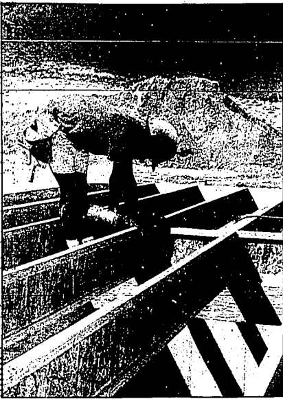
Engineered lumber can help keep a floor from squeaking.
