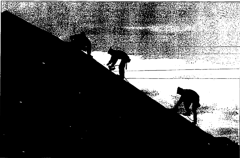
Roofers from Smith Roofing of Twin Falls place shingles on a house in the Candlridge housing development off of Eastland Drive. Density of residential development in some parts of the city's area of impact has drawn opposition from some neighbors.
