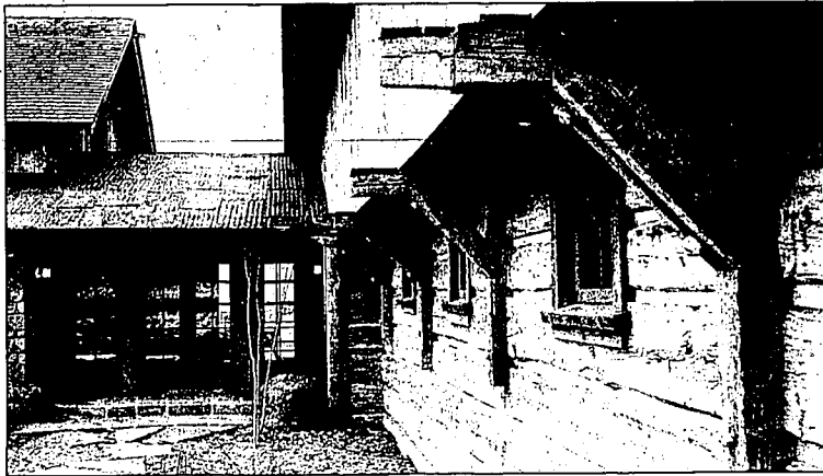
Timbers and wood recycled from older structures make up the exterior of a home in Bozeman, Mont., Nov. 17.
