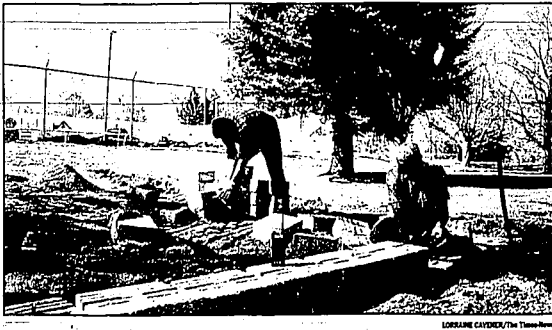
Raymond Alexander and Aaron Aggeler install a retaining wall for sand where a new playground will be installed at Shoshone City Park. The playground equipment is one of several new youth-oriented improvements in Shoshone Park.
