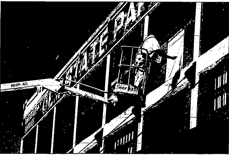
Gary Yetz, of Third Generation Painting of Twin Falls, paints a wood panel on the former Gem State Paper & Supply warehouse, which was built in 1918 or 1919, in Old Towne Twin Falls. Law, accounting and other financial-planning firms now occupy the building.
