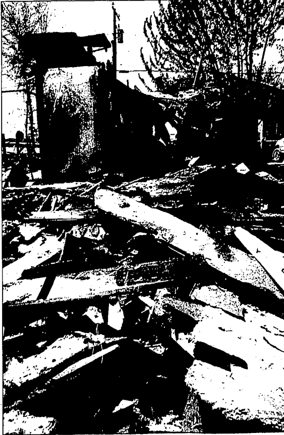
Three Twin Falls Fire Department engines and 11 firefighters responded to a fire at this vacant house on Ash Street over the weekend. There were no injuries, and the fire is under investigation as arson.
