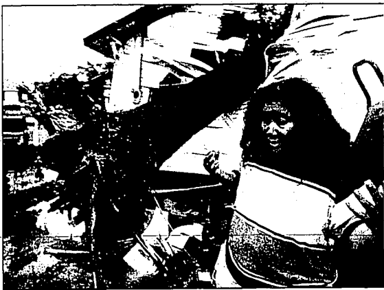
Roselyn Collins of Bryan, Texas describes what happened early Thursday when a severe storm caused a giant oak tree to fall through her home while she and her family were sleeping.
