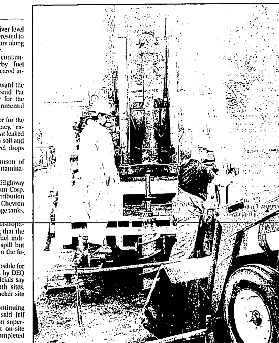
Gary Oylor and Ray Swensen of Hiddleston Drilling and Pump Co. drill wells at 425 E. Highway 81 in Burley as part of the ongoing cleanup of contamination from nearby fuel distribution centers.
