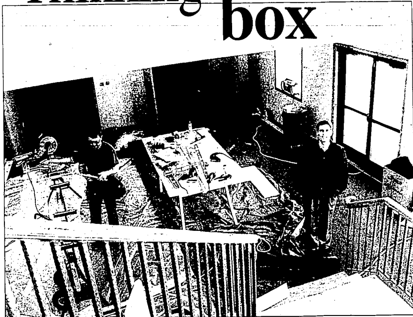
Pastor Dennis Stoneman stands in the entryway of the new multipurpose building at Burley's First Baptist Church. Nearby, a workman measures wood for cutting.
