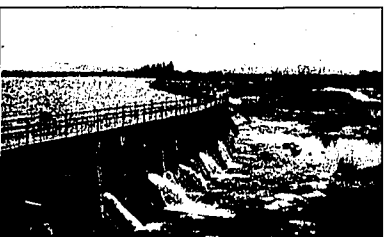
Water passes through the deteriorating spillway of Minidoka Dam, leading the Bureau of Reclamation to initiate studies into repair or replacement of the spillway.
