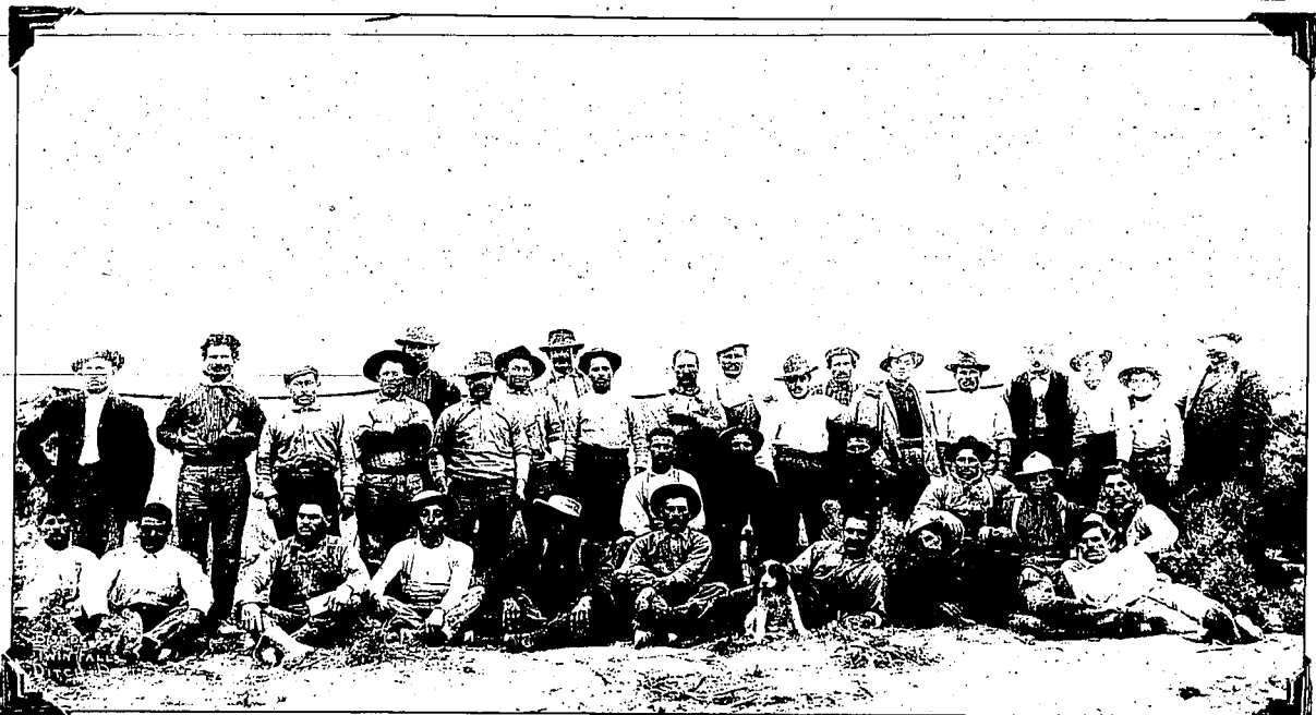
This image of ditch builders, labeled with the name of early Twin Falls photographer Clarence Bisbee, was recently scanned from a damaged glass plate negative in the Twin Falls Public Library's collection and restored by Blip Printers. Blip altered the photograph by moving and grouping the words which now appear in the lower left.
