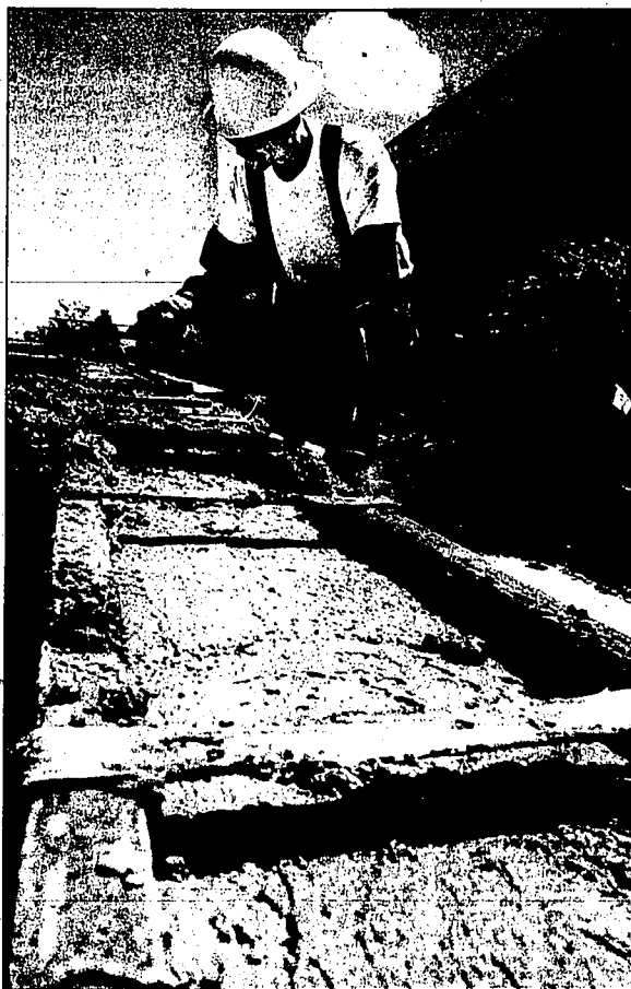
Mike Dehrie, with Peterson Brothers Construction Inc. of Twin Falls, on Friday smooths out the concrete of a stem wall foundation base for the Gold's Gym being built on Fillmore Street in Twin Falls.
