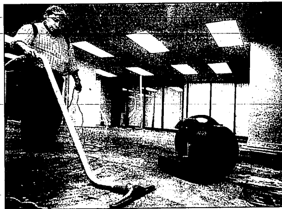
Marcos Morales works on cleaning up the mess at the State Capitol on Tuesday in Boise. A flash flood on June 29 displaced 20 workers and left 4,000 square feet of office space and the Legislative library at the State Capitol in need of $70,000-$100,000 of cleanup work.
