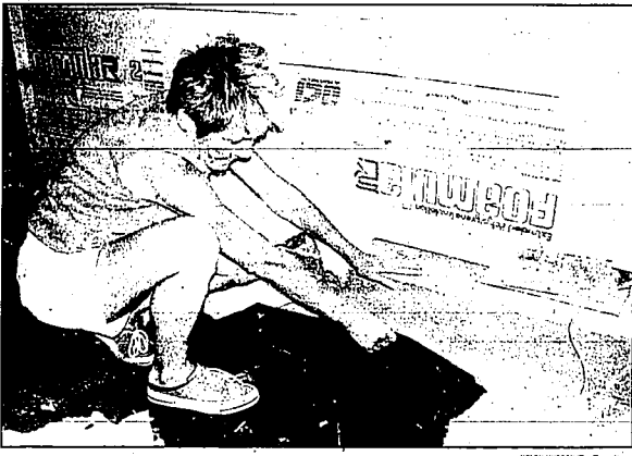
Radon inspector Mary Fisher discovers plastic not properly affixed to the foundation of a high-end home north of Ketchum. The plastic must be sealed tightly to the foundation to keep radon gas from entering the home.
