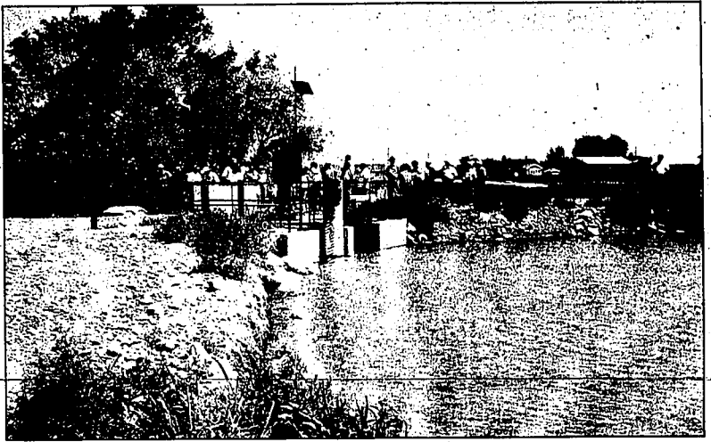
Britt Pond is an example of how canal companies are changing to meet today's concerns. This constructed wetland will serve a dual purpose: removing sediment and nutrients from irrigation return flows and providing irrigation water to subdivisions.
