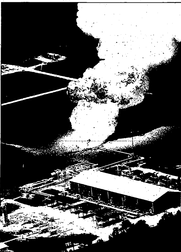
A gas explosion at the Duke Energy Moss Bluff storage site early Thursday forced dozens to evacuate near Moss Bluff, Texas, as an underground gas storage tank at the facility exploded and continued to burn.
