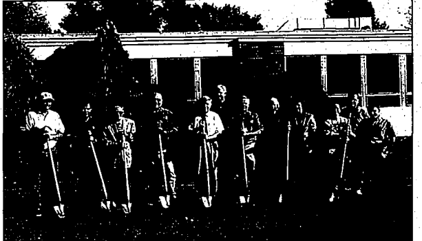
Minidoka Memorial Hospital in Rupert kicks off its construction project. The remodeling should take about nine months and will include new energy-efficient windows, a new roof, a new entrance to the Extended Care Facility wing and other improvements. From left are Garth Baker, hospital board member; Ted Garcia, chairman of the finance committee; John Cameron, chairman of the board of trustees; Dave Tester, chairman of the hospital board; Mark Newman, chairman of the construction committee; Carl Hansen, hospital administrator; Kathy Gonnell, Social Services; Teresa Hart, director of nursing in the Extended Care Facility; Jackie Hinrichs, activities director of Extended Care; Joel Rogers, human resources manager at Minidoka Memorial; and Dr. Kerry Saurey, medical director of the Extended Care Facility.
