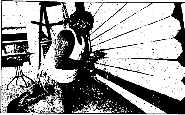
Tom Mignone boards up the windows of his restaurant, Breakfast at Lily's, in Satellite Beach, Fla., Friday. Hurricane Jeanne is expected to make landfall on the eastern Florida coast this weekend.
