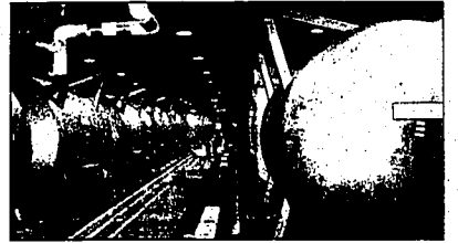
Giant containment cylinders that will be used to move deadly chemical weapons from storage igloos to an incinerator stand ready in this June 8 file photo, inside the Umatilla Chemical Weapons Disposal Facility outside Hermiston, Ore.
