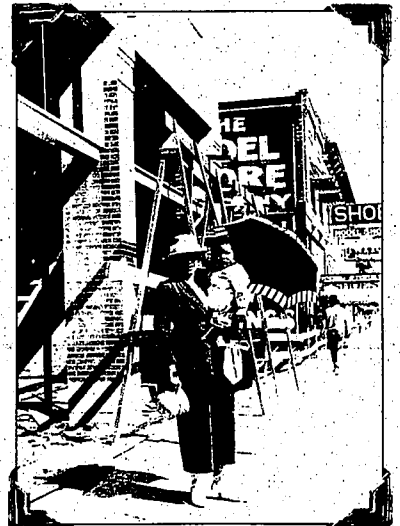
During Tom's Cafe construction in 1920, Kei Sakamakii Koto, wife of Tojiro "Tom" Koto, poses at the site holding their first son, Tom E. Koto, who was born in 1918 in Twin Falls. Kei was from the Saga Prefecture on Japan's Kyushu Island.
