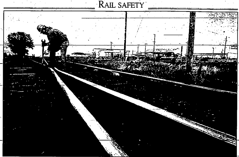
Mike Heath, a road master with Eastern Idaho Railroad, tightens bolts along railroad tracks in Twin Falls during a routine inspection Friday. As cooler temperatures descend on the Magic Valley, the steel rails contract and more of the bolts need to be tightened during inspections.
