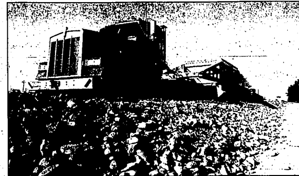
A belly dump truck unloads 18 of the 24,000 yards of structural fill that is being used to complete the sub-grade at the Lowe's construction site in Twin Falls on Monday. The home-improvement retailer plans to open its Twin Falls store in late 2005, creating about 175 jobs.
