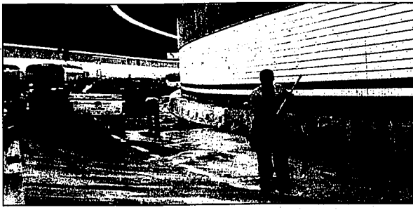
Workers clear water from the tunnel in the northbound lanes of I-93 in Boston file photo, after gridlock ensued when water began leaking into the tunnel, which carries Interstate 93 through downtown Boston. Boston's brand-new $14.6-billion highway tunnel has been found to be riddled with hundreds of leaks, and at least some of the problems were known to the builders back in the late 1990s.
