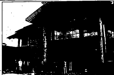
Construction workers are dwarfed by the new Dollar Mountain Lodge.
