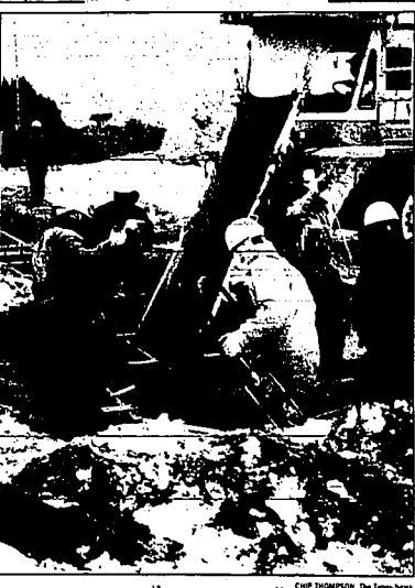
Workers for Lundahl Building Systems and Triple C Concrete pour footings for the Gossner Foods Inc. cheese factory at the Burley-Heyburn Industrial Park on Wednesday. Despite recent snow and daytime temperatures in the low 20s, Project Manager Scott Robinson said the construction is progressing on schedule. The plant is expected to begin operations by October 2005.
