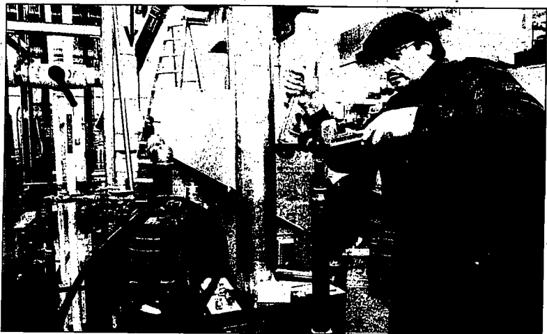
Ray Victoria, 42, of Marysville, Wash., assembles a hydronic heating system during a commercial/industrial refrigeration and heating ventilating and air conditioning technology class at Bellingham Technical College Dec. 8, in Bellingham, Wash.
