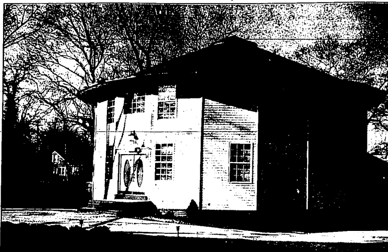
A suburban Washington family was definitely thinking outside the box when they designed this round house in Upper Marlboro, Md. Technically, the house is not a circle but a polyhedron made of 20 panels at 15 degrees.
