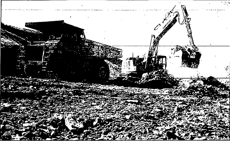
Crews move dirt into a truck at the Albion grade road project earlier this week. The $6 million project on Highway 77 between Junction and Albion is realigning the road to eliminate snow-drifting problems.
