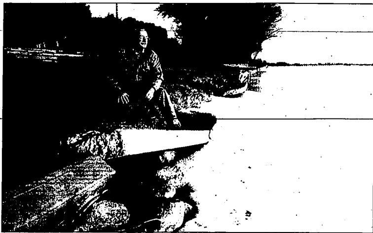
Bill Morrison kneels next to a retaining wall at his home along the Snake River near Hayburn. Morrison says the wall is breaking due to the pressure from ice, and he and several neighbors would like Idaho Power Co. to lower the river's water levels temporarily to give them time to make repairs.
