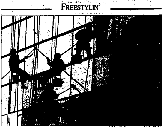
Workers hang from ropes to clean the glass walls of a skyscraper in Xi'an, in China's Shaanxi Province, Thursday.
